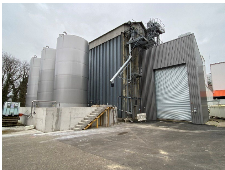
The Graines d'Alliance soybean crushing site in Saint-Sever (40)
